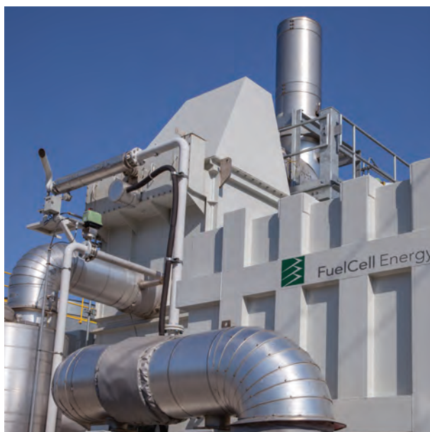
FuelCell Energy plant in Bridgeport, Connecticut.
