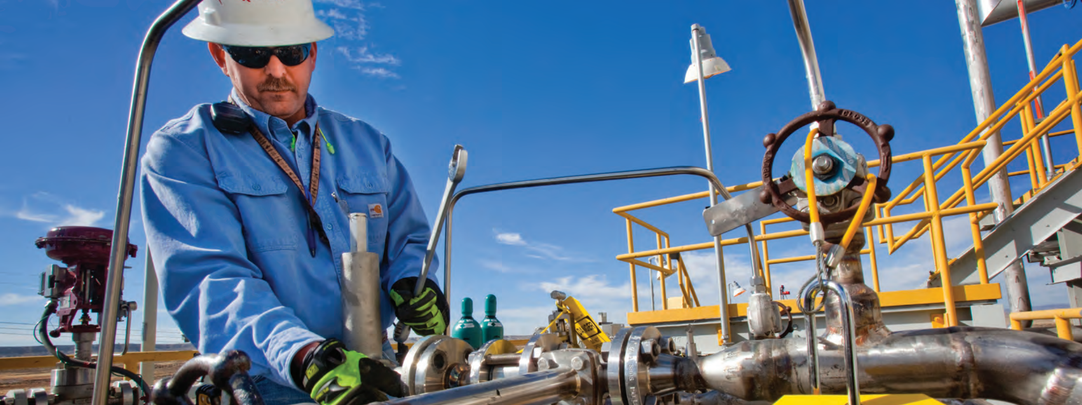
Heath Eddins, facility plant superintendent, inspects equipment at our LaBarge gas plant in Wyoming.
